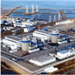
Image Haiyang nuclear power plant. Photo credit: State Power Investment Corporation.
