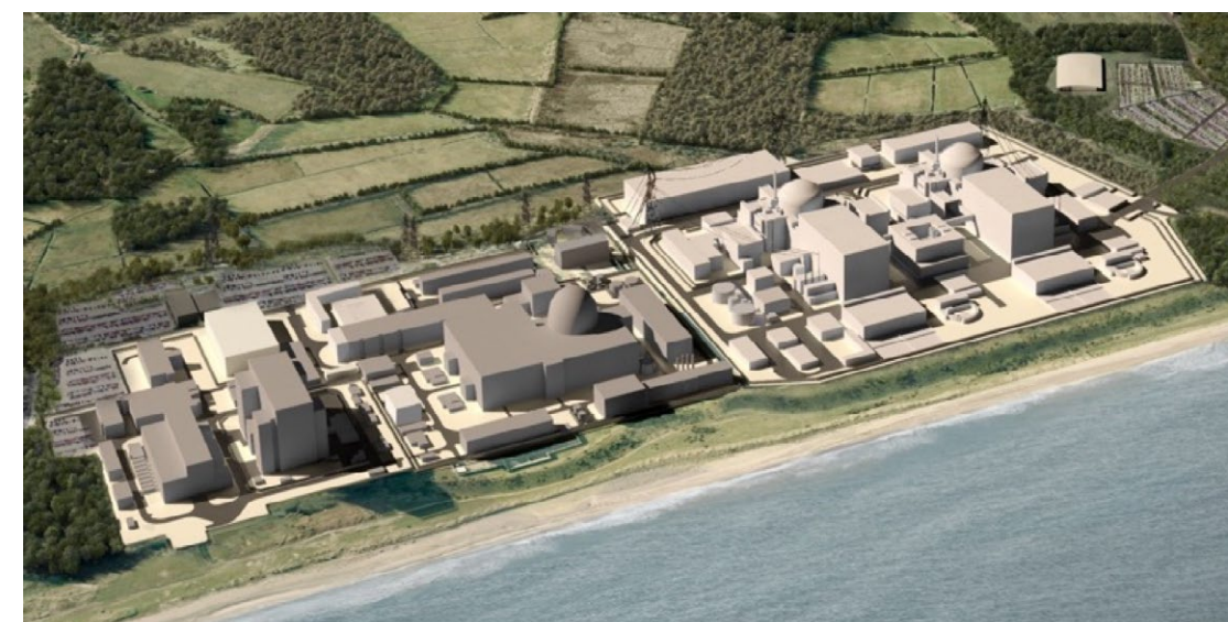
Image Proposed Sizewell C nuclear power station. image credit: EDF Energy.
